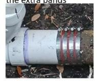
This is a pipe hanger used to carry the pipes under your slab. Why? Because the backfilled dirt will settle over time
